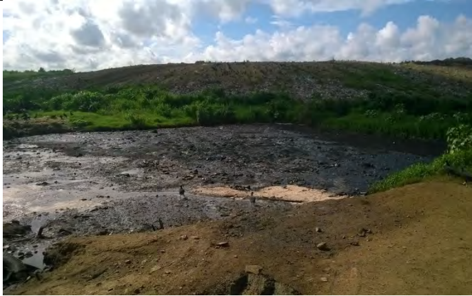
Figure 5.13 The 1 st receiving pond at the Beetham FSTF filled with dried FS
