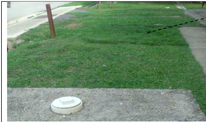
Figure 5.2 A septic tank and soakaway system
